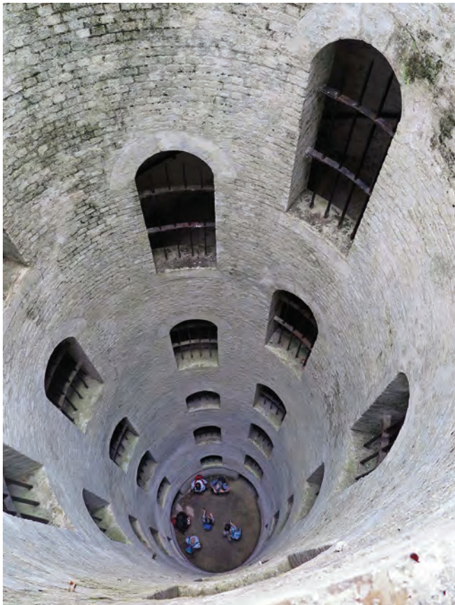
The light well of the Grand Shaft showing three spirals of 'borrowed lights' that illuminate the stairs.
